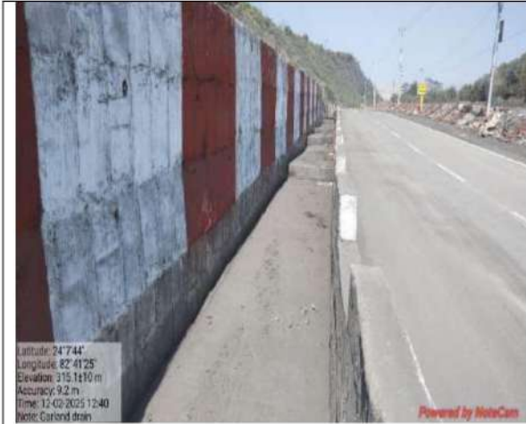
Pic 1:- Drain Besides OB dump
